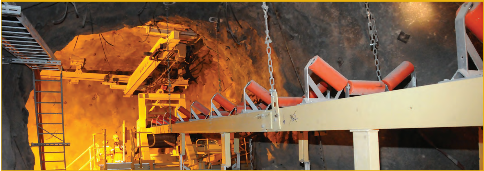
Underground conveyor, Chelopech
