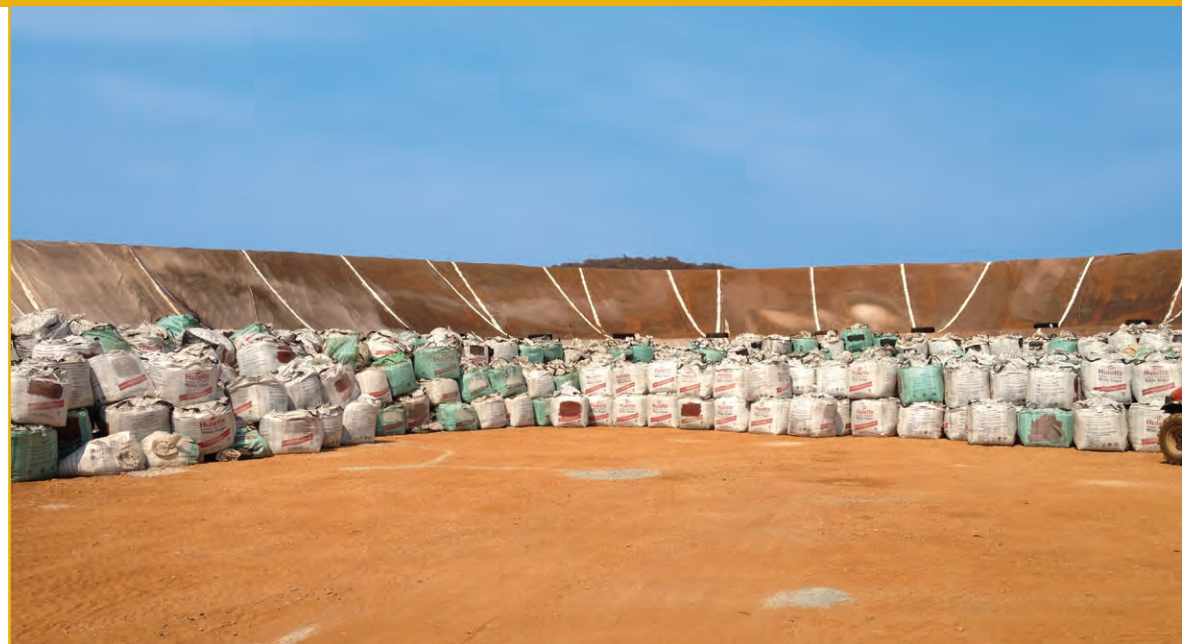
Hazardous waste facility, Tsumeb
